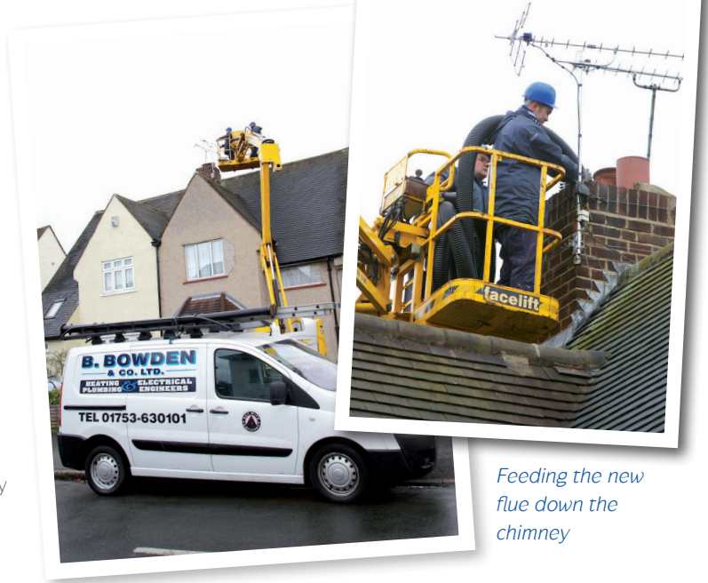
Getting ready to remove the old flue
