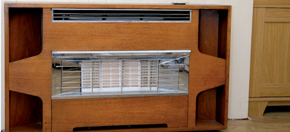
Before removal of the old back boiler and gas fire
